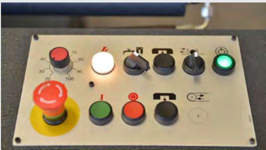
PIC.: CONTROL PANEL
